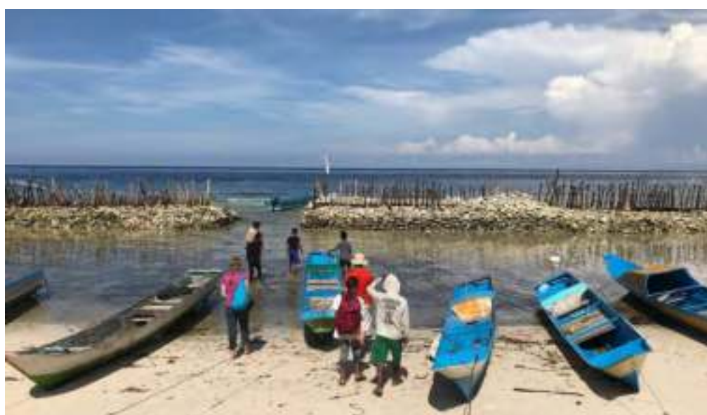
Figure 12. Sea wall in front of village to avoid big waves and floods into the village
