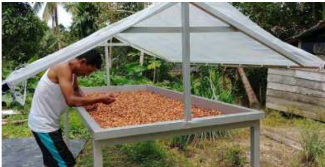
Figure 12: A cacao drying house in Masihulan provided by as part of a government program
